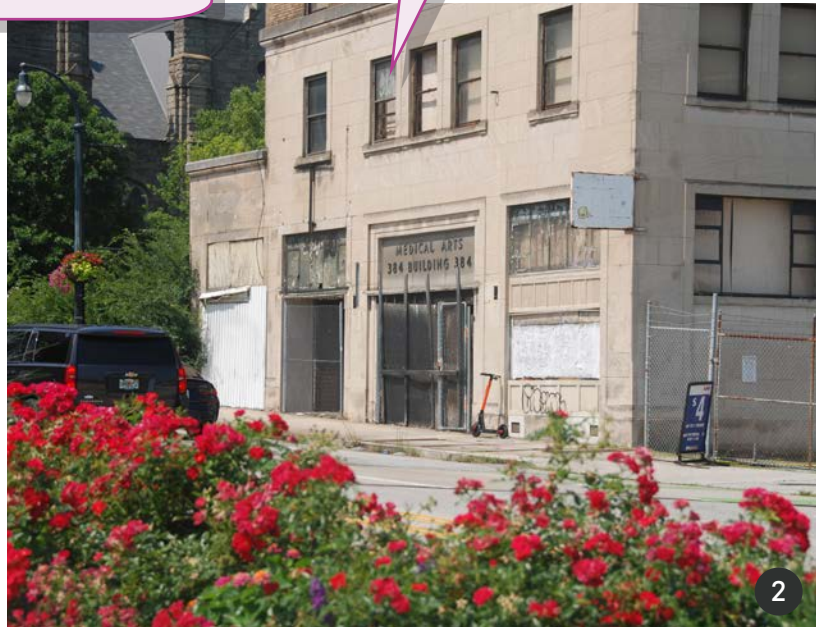
1) Bridge over the Connector 2) Vacant Medical Arts Building
